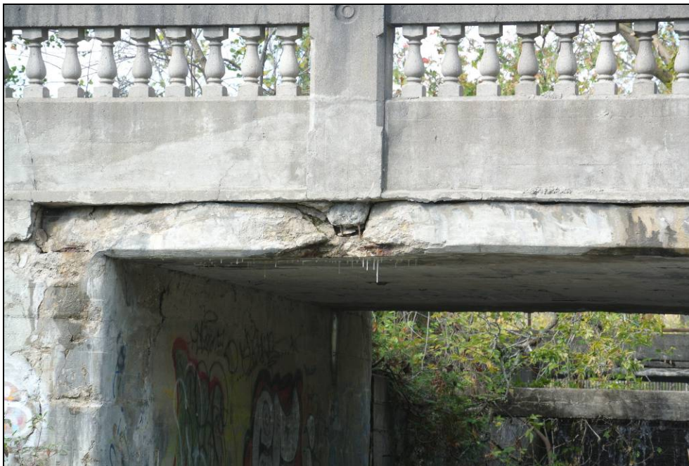
Plate 14: Detail of soffit, east railing system, and south abutment.
