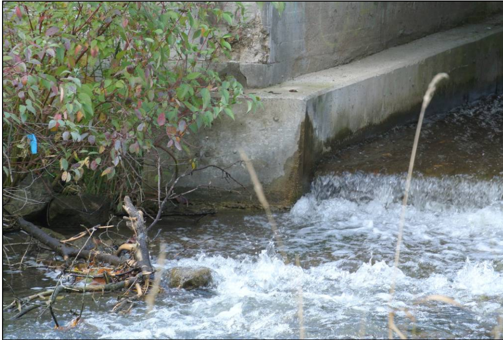
Plate 17: Detail of the footings on the southeast corner of the south abutment.
