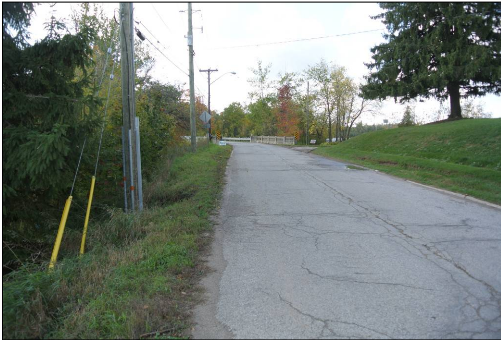
Plate 1: North approach to the bridge.
