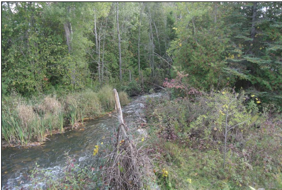
Plate 20: Spillway to the east of the subject bridge, looking northeast.
