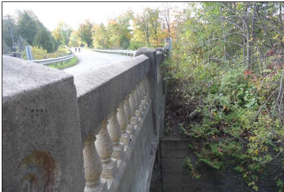
Plate 7: Oblique view of the west elevation, looking south.
