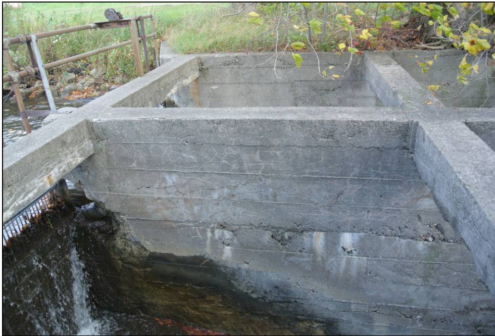
Plate 19: Detail of stop log control structure.
