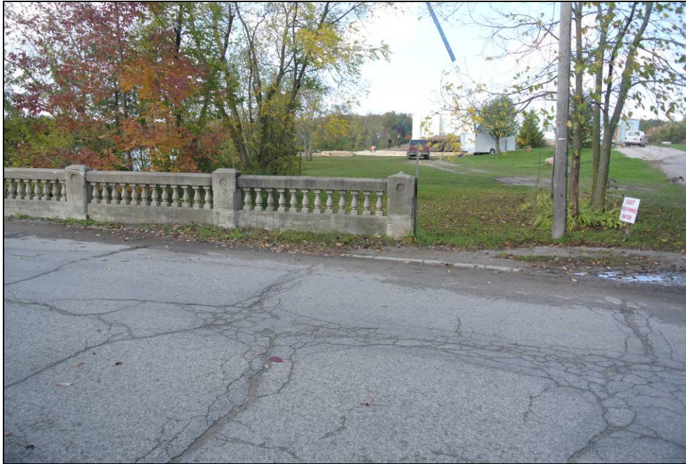
Plate 9: View of concrete railing system at the northwest corner of the bridge.
