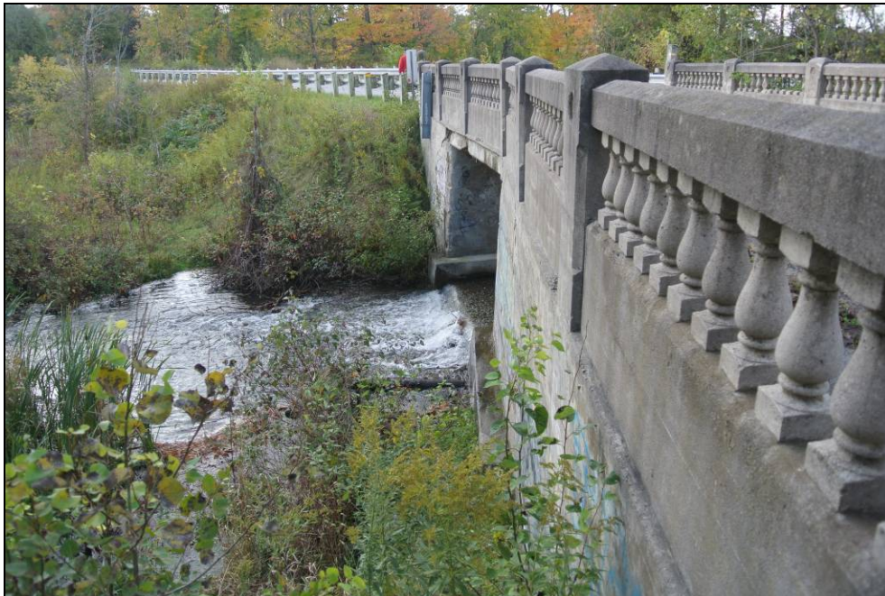
Plate 6: Oblique view of the east elevation, looking south.
