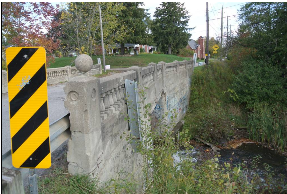
Plate 4: Oblique view of the east elevation, looking north. Note the spherical adornment on the southeast endpost of the railing system.
