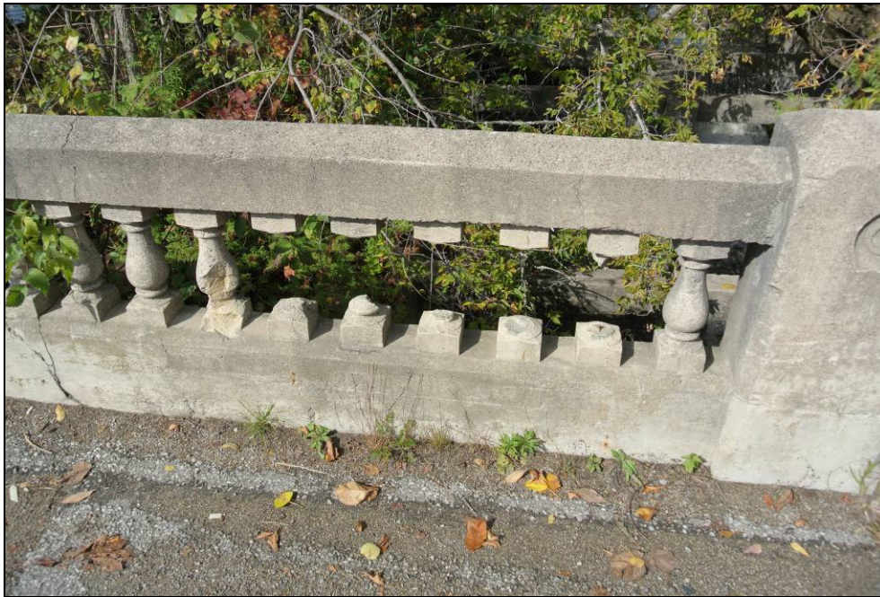
Plate 13: Detail of concrete railing system with spindles removed.
