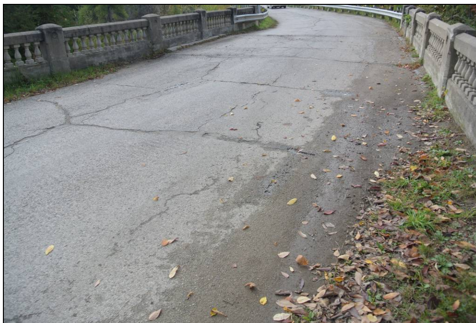
Plate 8: View of the bridge deck, looking south. Note the concrete railings with spindles lining the asphalt deck.
