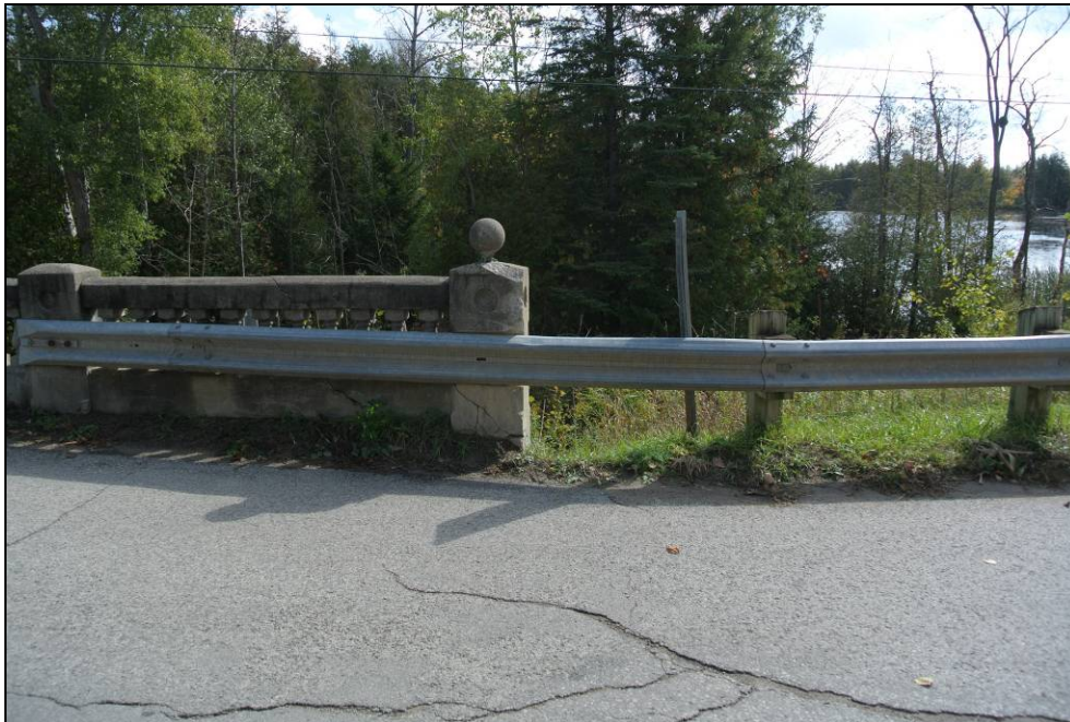
Plate 10: Detail of steel barrier attached to the concrete railing system at the southeast corner of the bridge.
