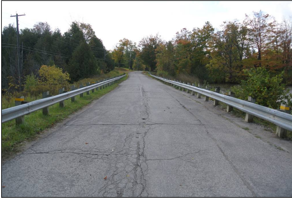
Plate 21: View along the Hillsburgh Dam to the south of the subject bridge.
