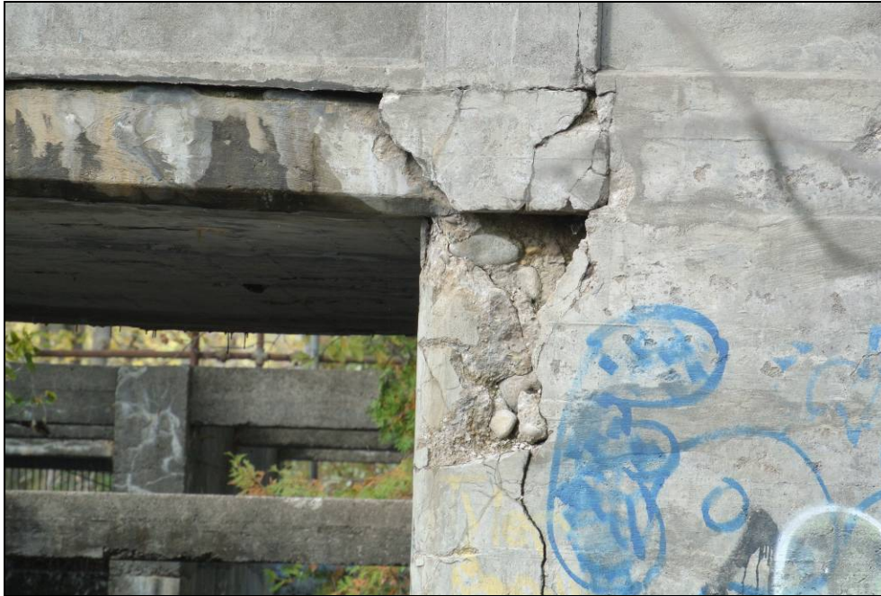
Plate 15: Detail of concrete deterioration at east side of north abutment.
