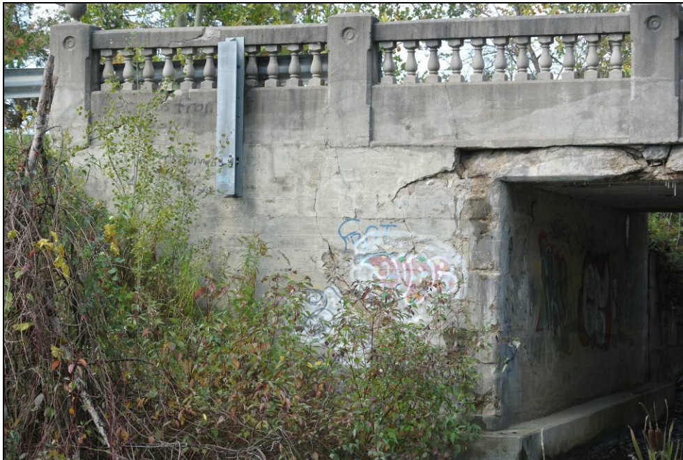
Plate 16: View towards east side of south abutment.
