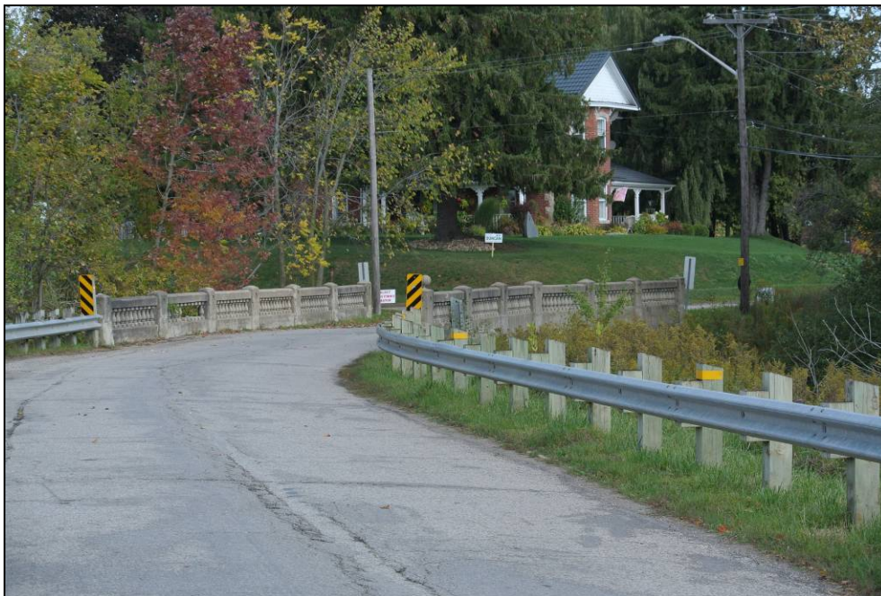
Plate 2: South approach to the bridge.
