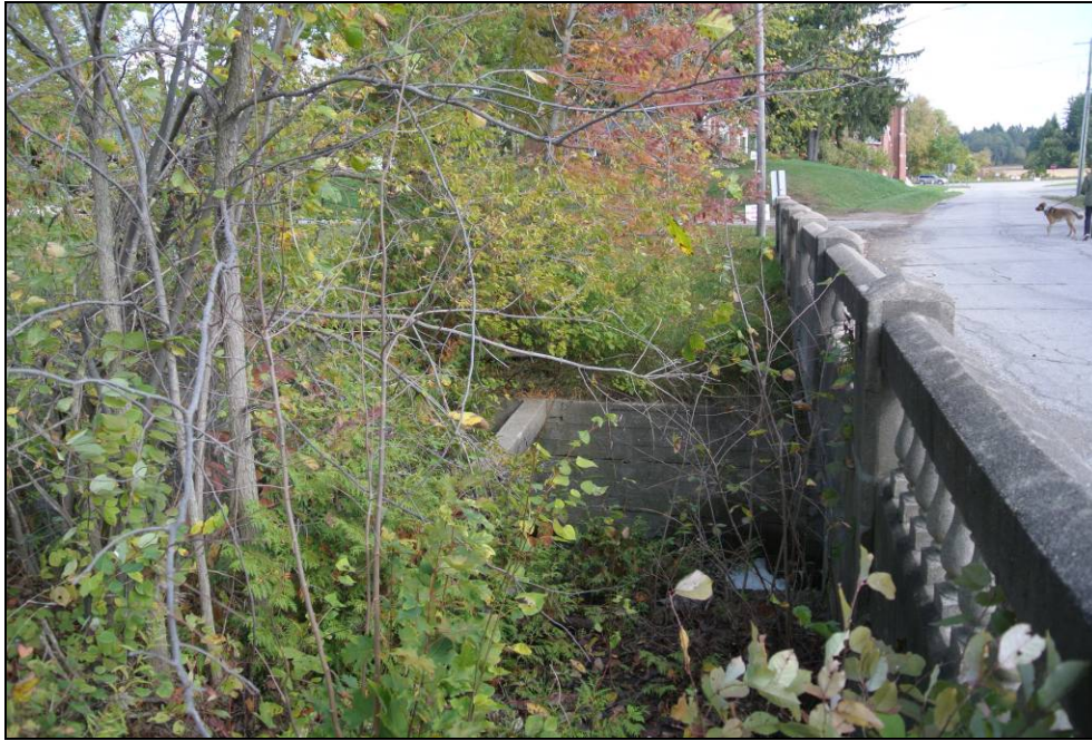
Plate 5: Oblique view of the west elevation, looking north.
