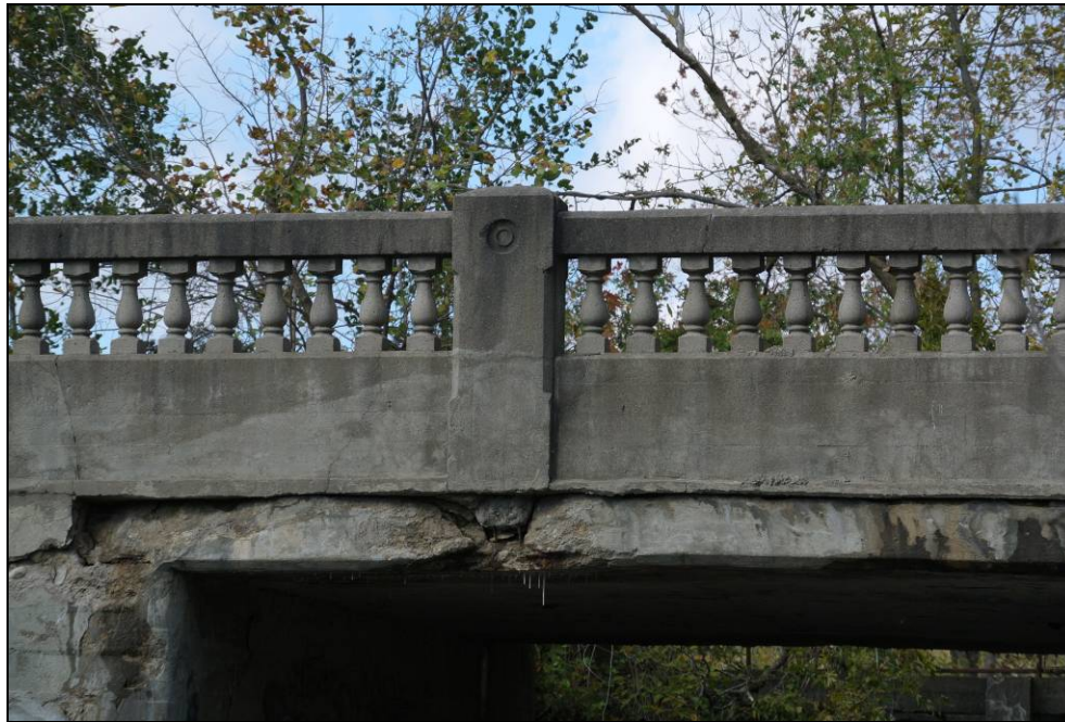
Plate 11: Detail of east side of east railing.
